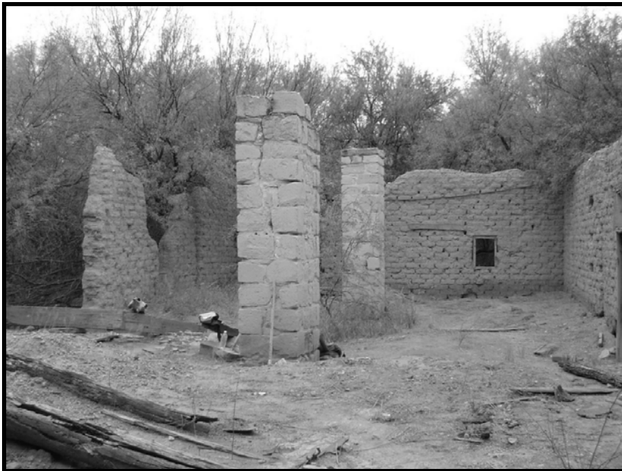
The remaining adobe walls of the Munguia homestead as they look today. Photograph by Jacquie Dale.
